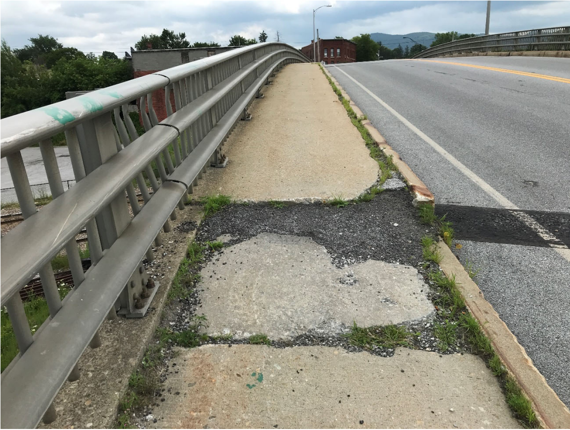
Sidewalk and Guardrail.
