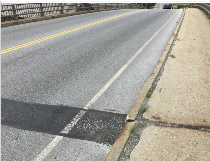
Deck center span
