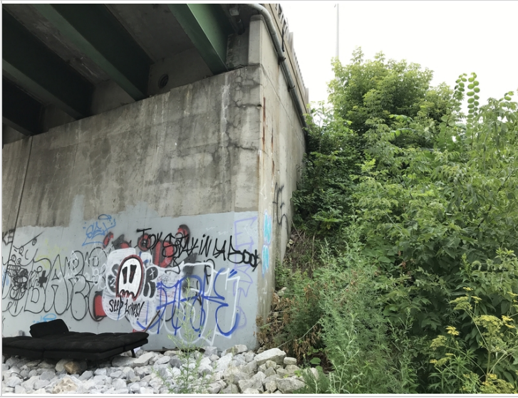
NW retaining wall
