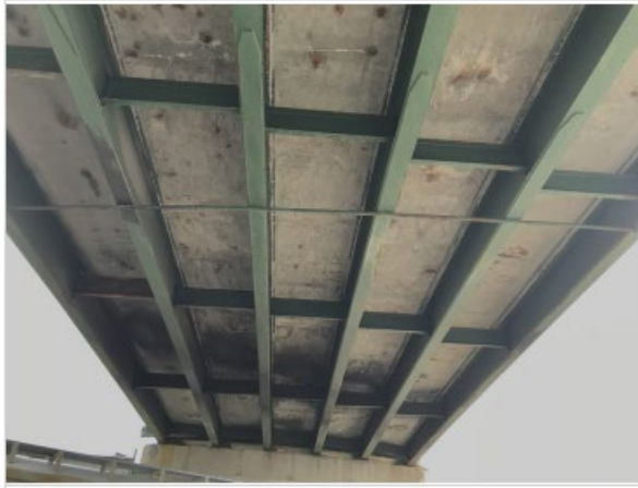
Center Span East pier
