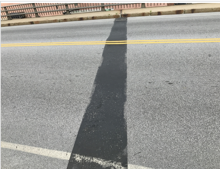
Joint East pier
