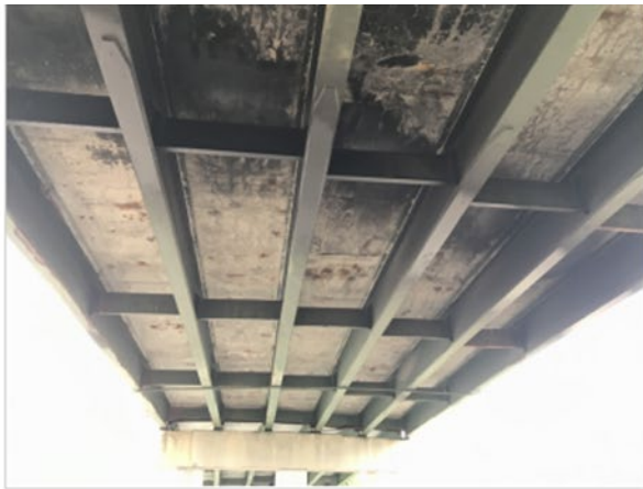
Center span West pier
