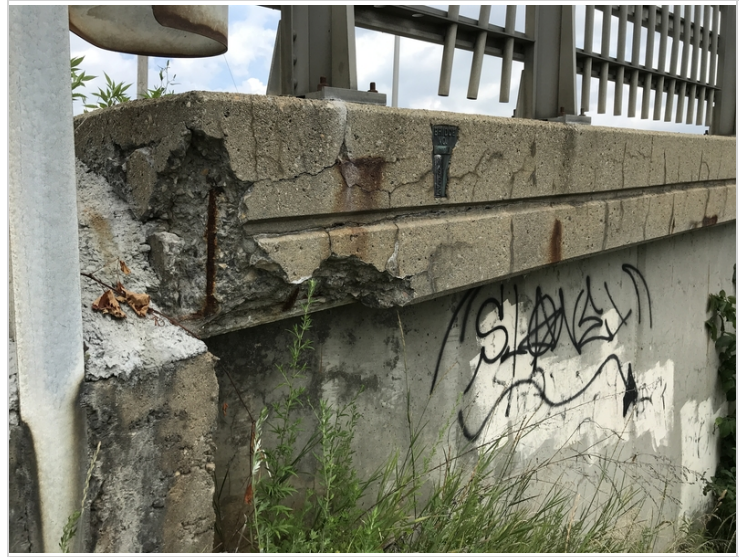
SW end approach curb/fascia
