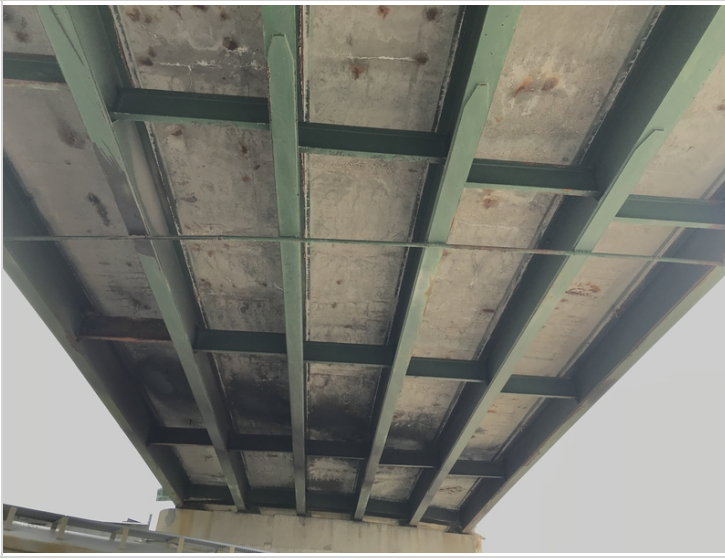
Center Span East pier
