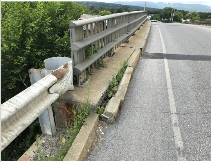
South curb East end
