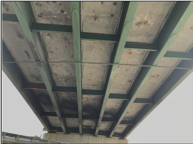
Center Span East pier
