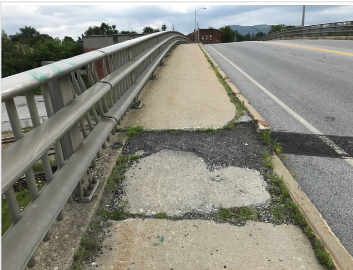
Sidewalk from West abutment
