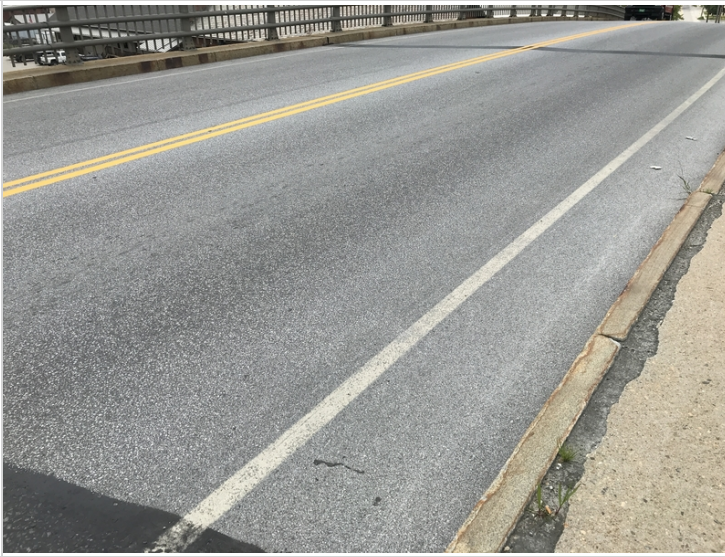
Deck East span
