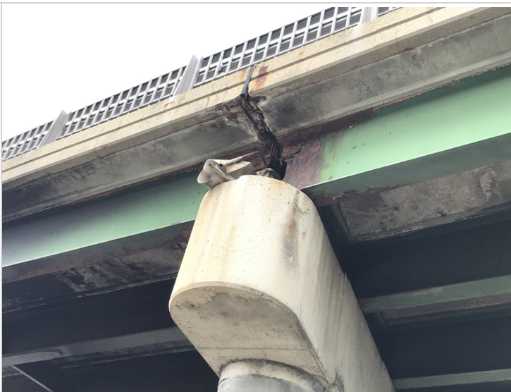
South end East pier joint
