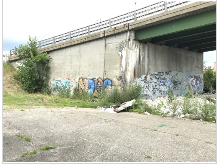
SW retaining wall
