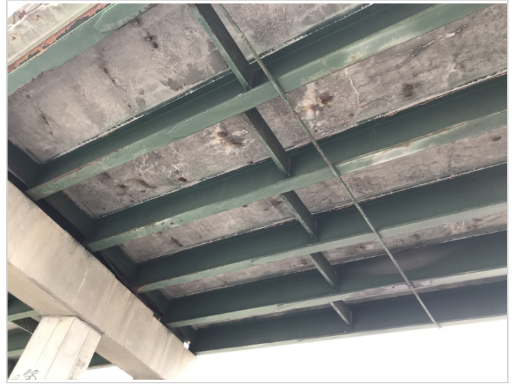
Center span West pier
