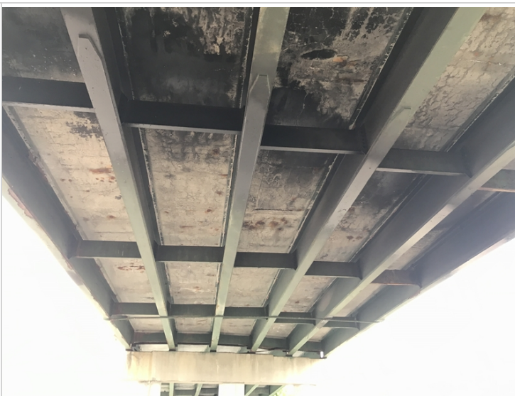
Center span West pier
