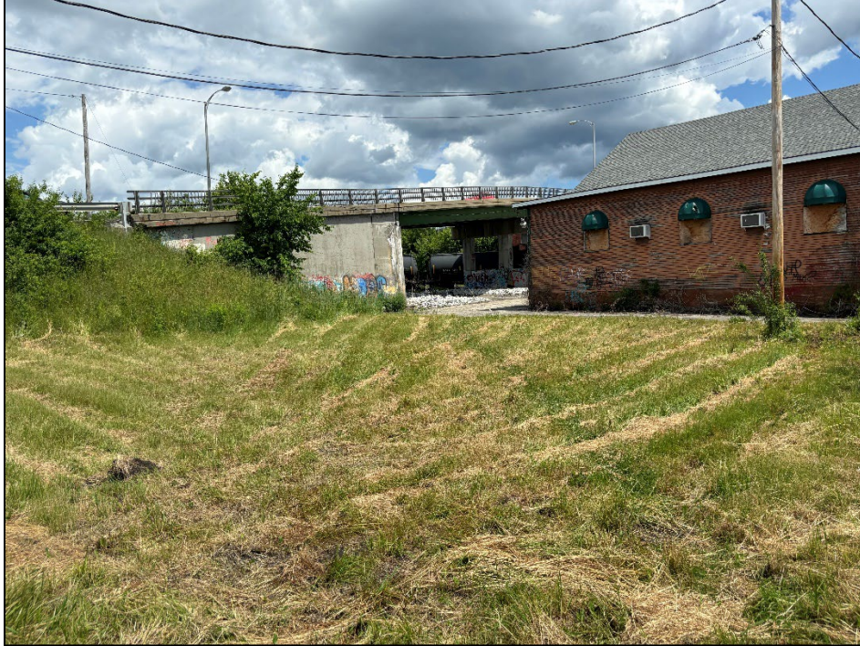
Figure 5. Overview facing northeast towards River Street with depot and flattened land.
