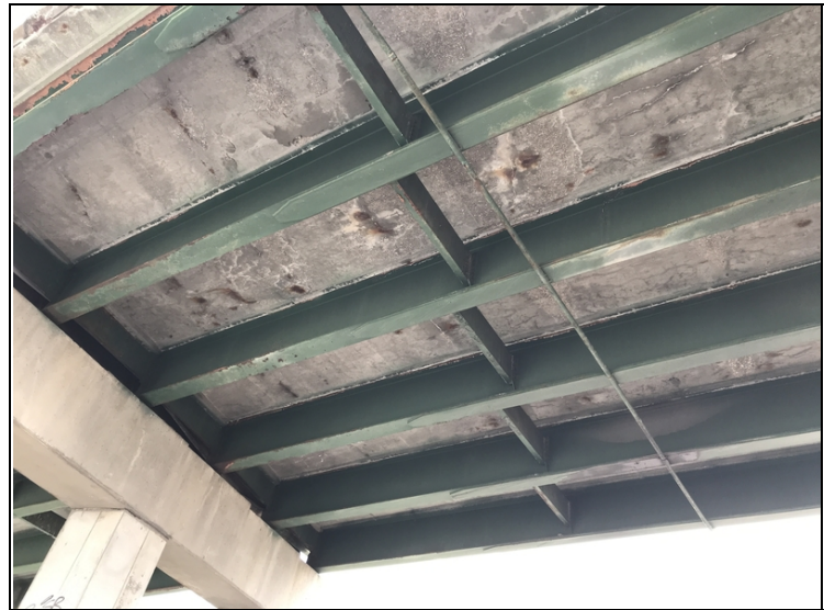
Center span West pier
