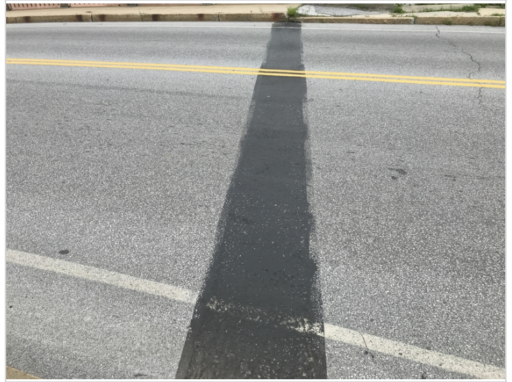
Joint East abutment
