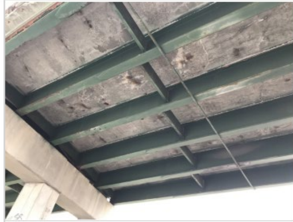
Center span West pier
