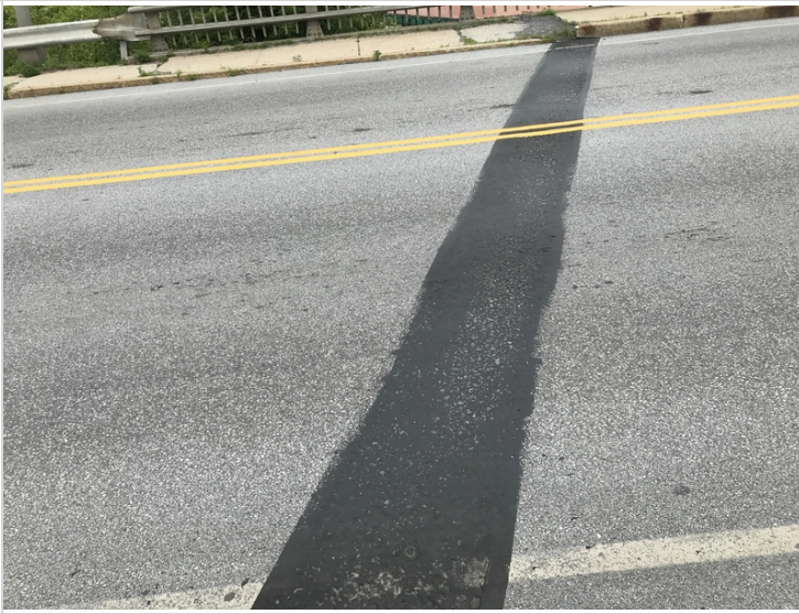
Joint West abutment
