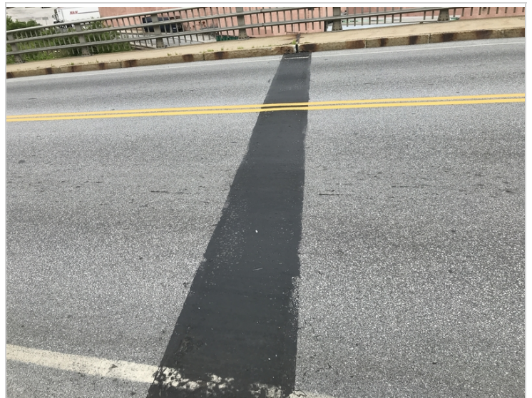
Joint West pier
