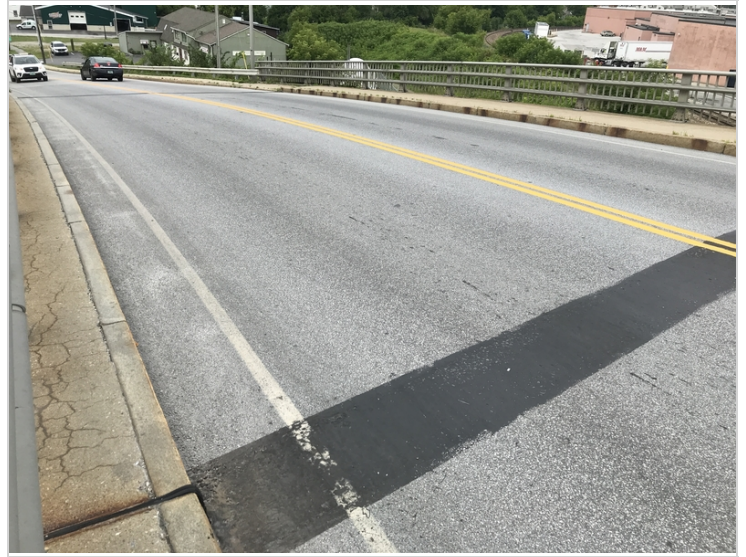
Deck West span
